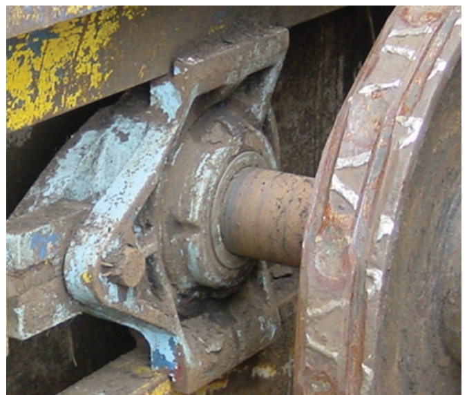
Cooper tension take-up unit in a trapped location on a sugar mill conveyor
